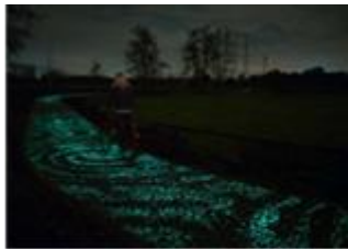
Figure (19): The smart road stores energy during the day and then glows during the night
