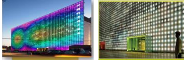
Figure (24): Advanced Curtain Wall System developed by adding photovoltaic cells to curtain 8
