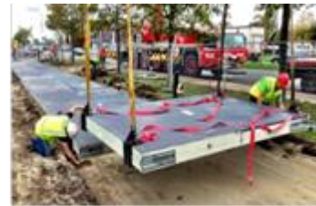
Figure (21): Modules of silicon crystalline solar cells, which are combined with a concrete layer.
