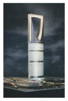
Using glass facades, which do not meet the climate requirements in Saudi Arabia
