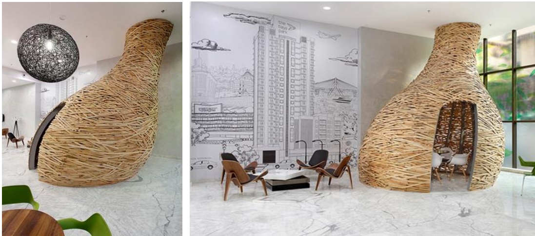
Figure (5) - The nest is constructed from a curving frame of plywood ribs that narrows as it approaches the ceiling and is clad in strips of pine salvaged from inside shipping containers. Its organic form provides a sculptural presence in the lobby, while the woven surface lets daylight from the adjacent windows filter into the interior. https://inhabitat.com/planet-3-studios-weaves-nest-like-meeting-space-with-recycled-pine-wood-strips/
