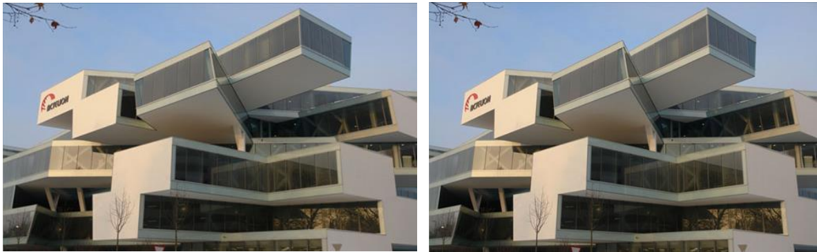
Figure (21) - each of the six floors has a unique footprint and many hang seemingly impossible lengths over the floors below them. These unique floor plans create open spaces for green roofs on the third and fifth floors to encourage comfort and provide green space for stifled employees.
