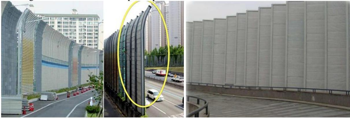
Pic. (1-2) Shows using noise barriers to reduce noise.
