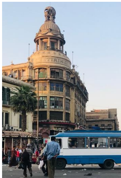
Figure (4), Tiring building with neo-baroque style(source: the authors)
