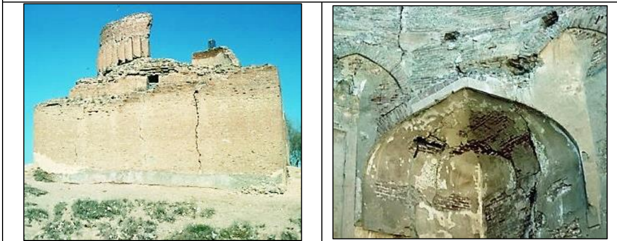
Plate (7) shows the exterior and interior of Ardabil dome (Archnet) 118
