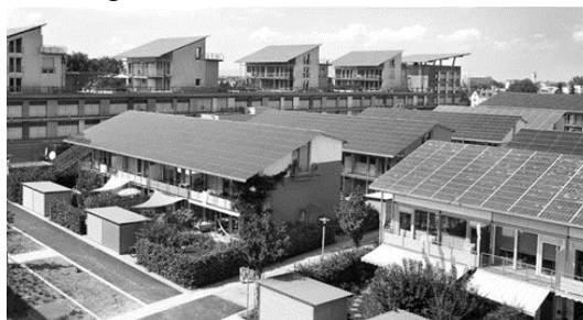
Figure (3). The Solar Settlement, a sustainable housing community project in Freiburg, Germany. (Adopted from: https://en.wikipedia.org/wiki/Photovoltaics#Overview )
