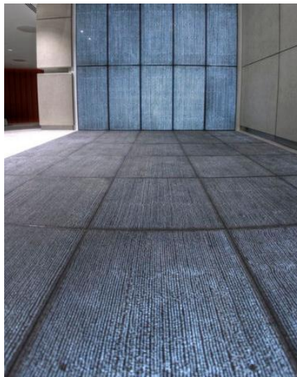
Figure 12 the first time to use transparent concrete in flooring in London & Oriental's London offices – features
