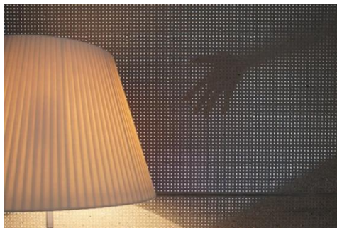
Figure 7 the application of transparent concrete panels in form of a partition wall in “Europe Point”
