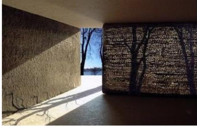
Figure 6 using the translucent concrete in Walls
