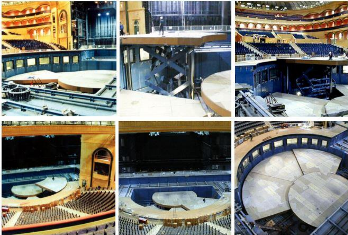
Fig 26, Cirque du Soleil show, "O". stage platforms featuring custom underwater lifts
