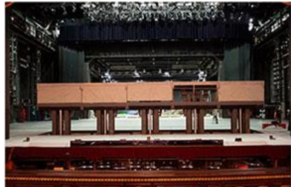
Fig 14 All platforms and mechanisms move silently, smoothly, their speed can reach 0.5 meters per second
