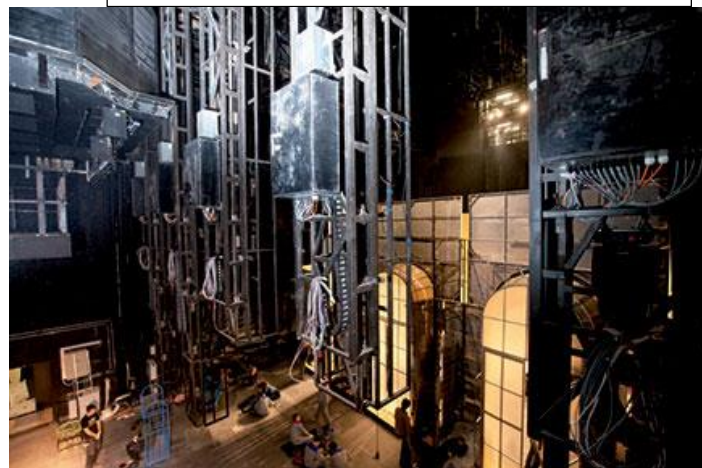
Fig 13 the light bridges in the main stage which moves vertically and horizontally
