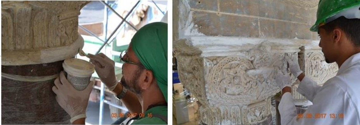
Fig (20) Integration of the missed parts of stucco decorations
