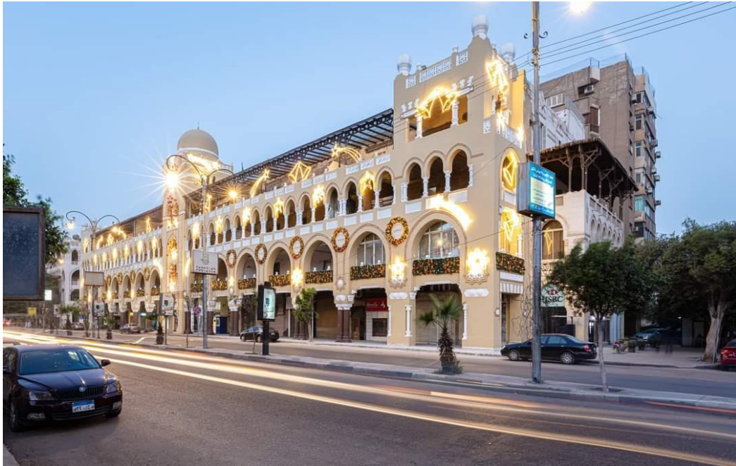
Fig (23) the front facade after restoration
