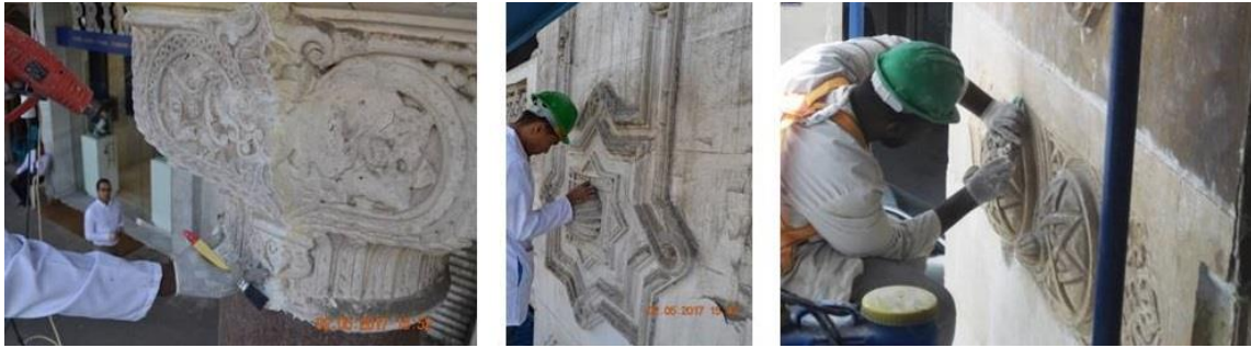
Fig (17) Mechanical Cleaning by using metal tools to clean the solid dirty that steamer couldn't remove it Integration injection and consolidation:
