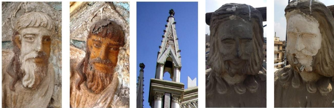
Fig (12) overprinting's layers by oil colors at Maronite Church
