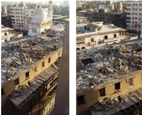
Fig (10) the buildings' roof covered by rubbish
