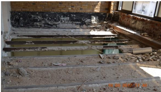
Fig (8) destroyed concrete ceiling because of transferring the balcony to swimming pool without isolating the floors
