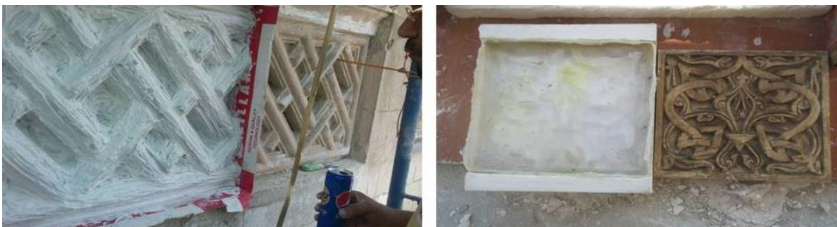
Fig (22) Silicon casting molds were made to parts that have fine decorations
