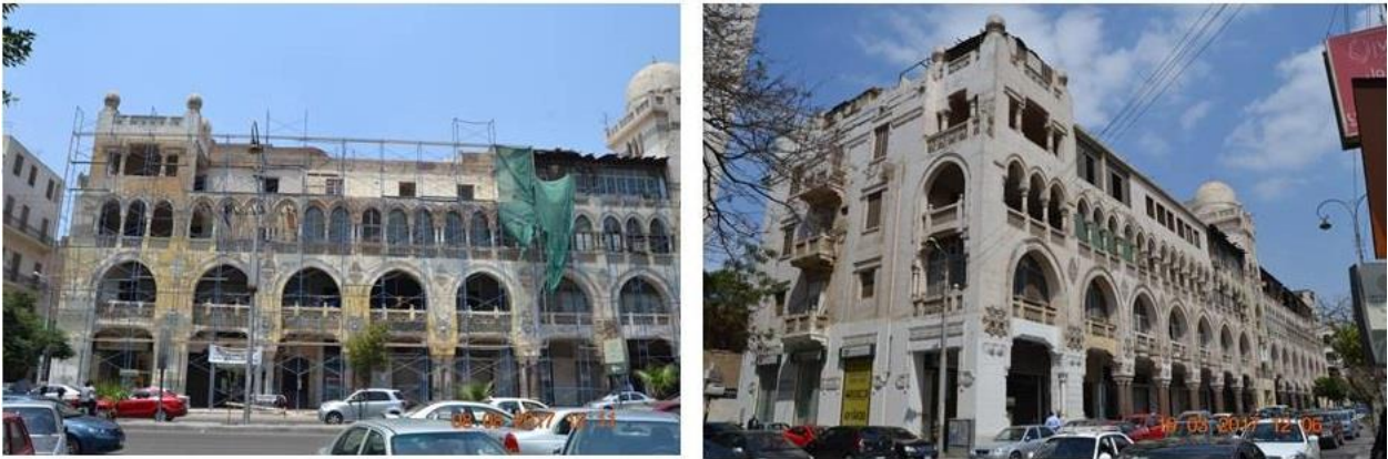
Fig (15) Removing the added parts to the original building
