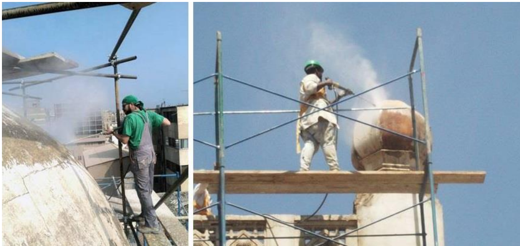
Fig (16) cleaning by steamer to remove the over paintings.
