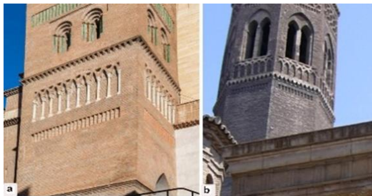
Figure 20. Blinded arcades of overlapping arches (a) San Bedru church, Teruel. (b) San Bablo church, Zaragoza; Guzman, 2003.
