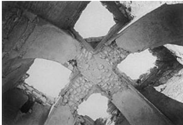
figure 5. two cross-arches roofed a room in al-kharana palace; al-kadi, 2016.
