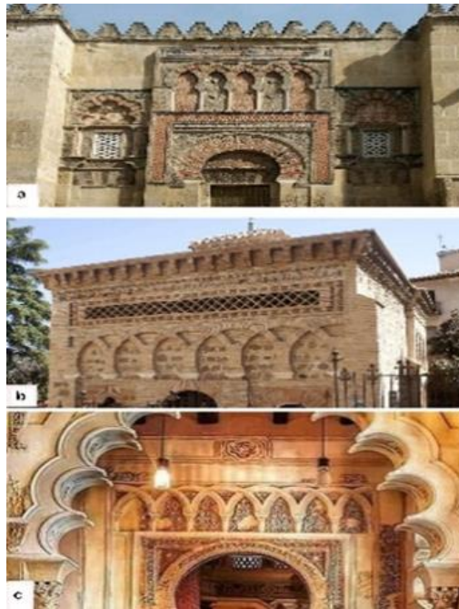
Figure 10. Blinded arcade of overlapping arches (a) San-Estiban gate, Cordoba Mosque; Khoury, 1996. (b) Bab Mardoum mosque, Toledo; King, 1972. (c) Ja'faria mosque, Zaragoza; Bloom, 2020.
