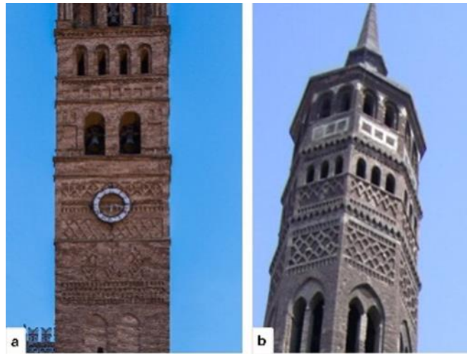
Figure 19. Decorations of overlapping arches in cathedral's towers (a) Tarazona cathedral, Zaragoza. (b) San Pablo church, Zaragoza; Fuentes, 2013.
