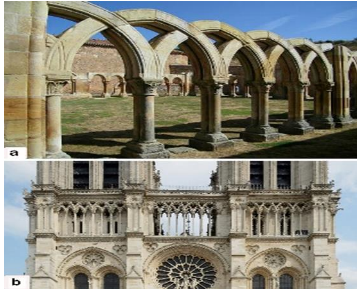
Figure 22. Arcades of overlapping arches in European architecture (a) Monastery of San Juan de Duero in Soria, Spain; Garsía, 2015. (b) Notre Dame cathedral, Paris; Bruzelius; 1987.
