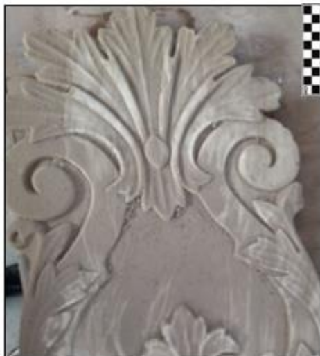
Figure 14. During mechanical cleaning of the marble decorative unit
