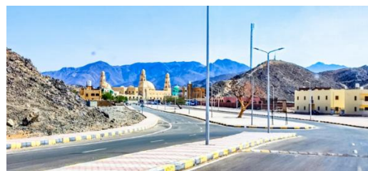
Fig.6 section c-c -Village entrance) source: (source: photograph by the author)
