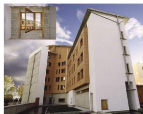
Fig (27 b) French Regional Government Office multi-story building using hemp block infill walls (Rachel Bevan and Tom Woolley, 2008).
