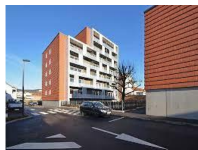
Fig (45) 7-storey modular building in France by Herbert Gruber [48].
