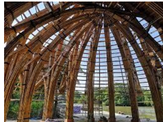
fig (19) Thailand-pavilion-bamboo build
