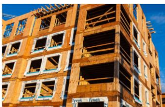
fig (6) Wood-framed apartment construction in Vancouver, Canada [3]
