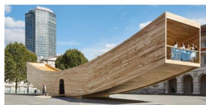
fig (7) Prefabricated smile building of 12 industrial-sized tulipwood, CLT panels by CLT pioneers, Züblin-Timber in Germany [4]
