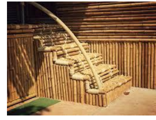
fig (20) Bamboo is used as stairs material
