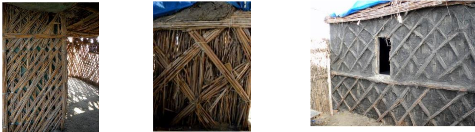
Fig (24) The usage of reed in forming vernacular buildings. (Marwa, 2015)
