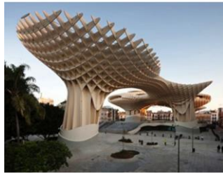
fig (16) Metropol Parasol Structure [16]
