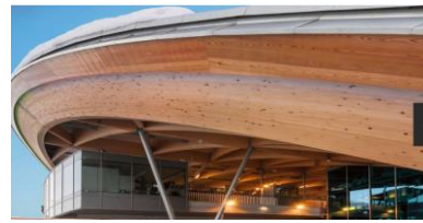
fig (8 b) Curved beam
