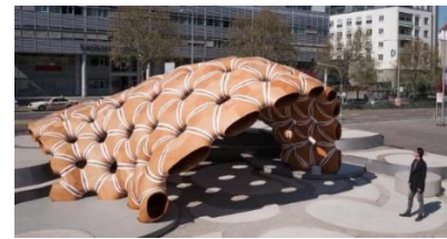
fig (17) Robots build sea urchin prefab pavilion using biomimicry [17]
