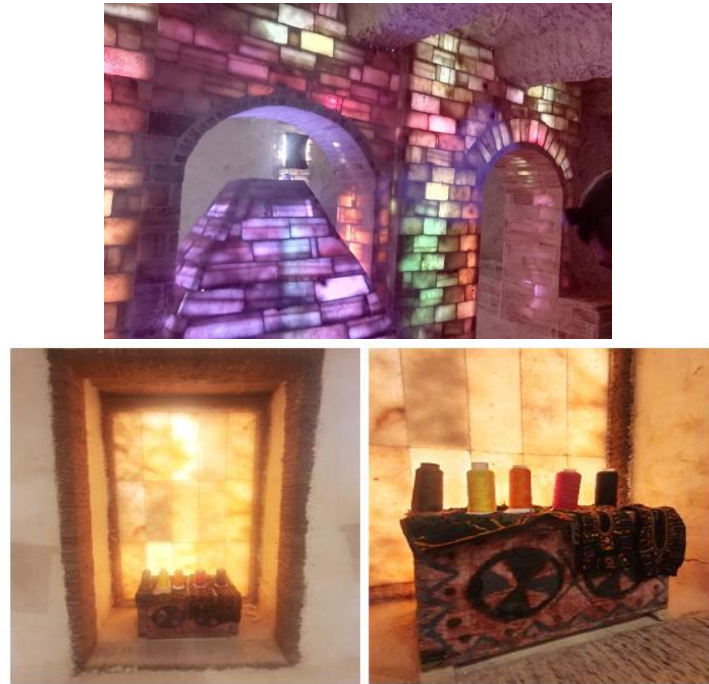
Figure 10: Siwa Museum - Salt Block Opening as an Alternative to Glass Bricks (Researcher, 2023)
