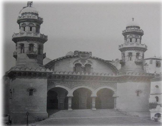
Photo No.01: The eastern facade of the cathedral (the cathedral in 1839 AD)
