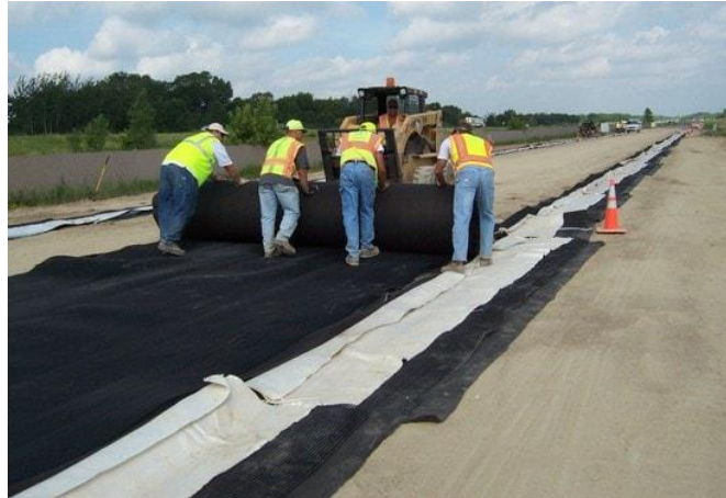
Fig (2): Geo-textile in road construction (19)
