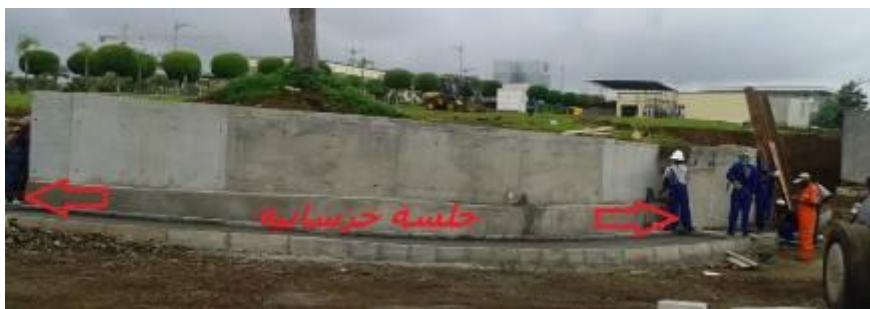
Fig. 6 the concrete mural involved in the research.
