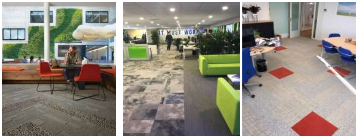
Figure (2) shows the use of synthetic carpets made of natural fibers from the sisal plant to cover floors in public places
