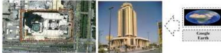
Figure 4. Aerial and field imagery via Google Earth for the site of the Municipal Palace Building.
