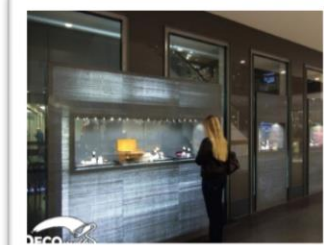
pic.2 shows the translucent concrete in the interior design.
