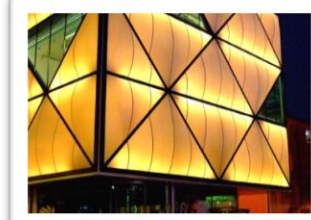
pic.5 shows ETFE panels on the buildings facades.
